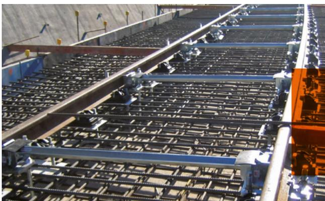
adjustment of a track panel with direct fasteners (Adelaide / Australia)
